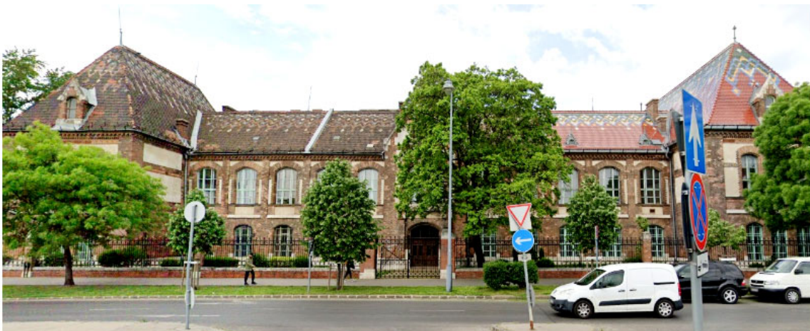
Figure 4: Image of MM-MG building [25]
