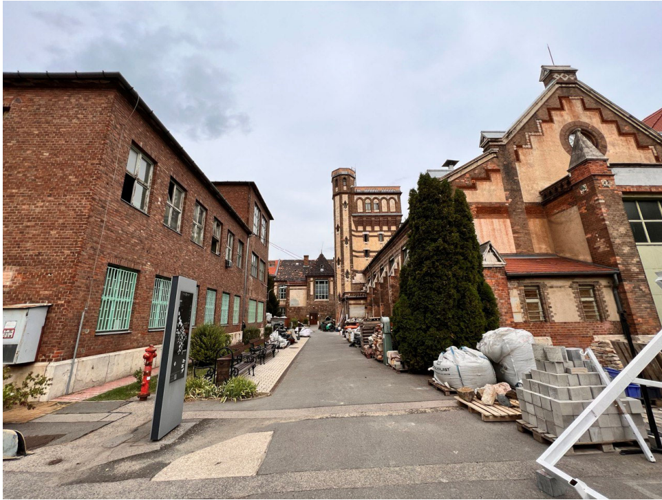
Figure 5: Another side of MM-MG building
