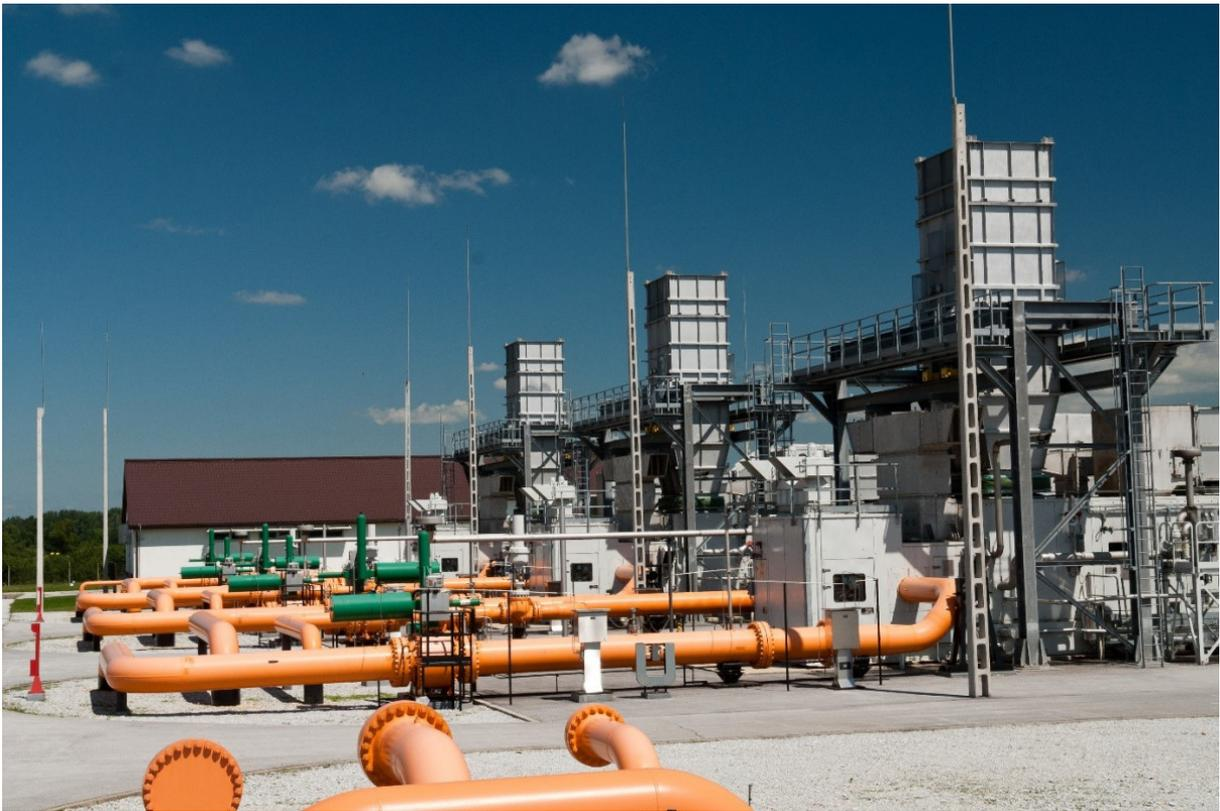
Figure 4.1: Compressor station [19]
