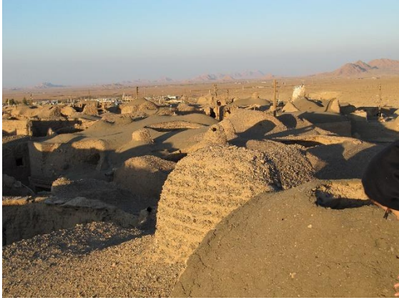
Figure9: roof of traditional houses with mud material, village of Mazar in arid climate source: author
