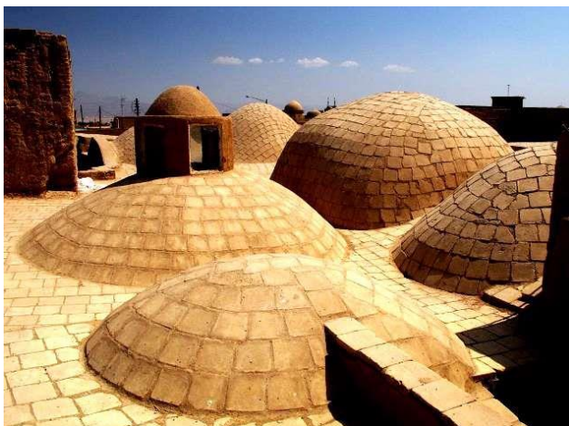
Figure 8: roof of traditional houses with brick material, source: www.dana.ir
