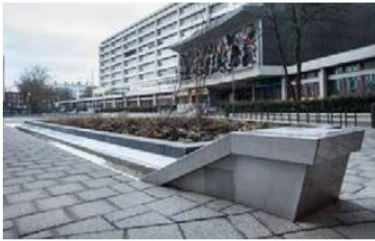
Functional storm water inlets are designed as special features
