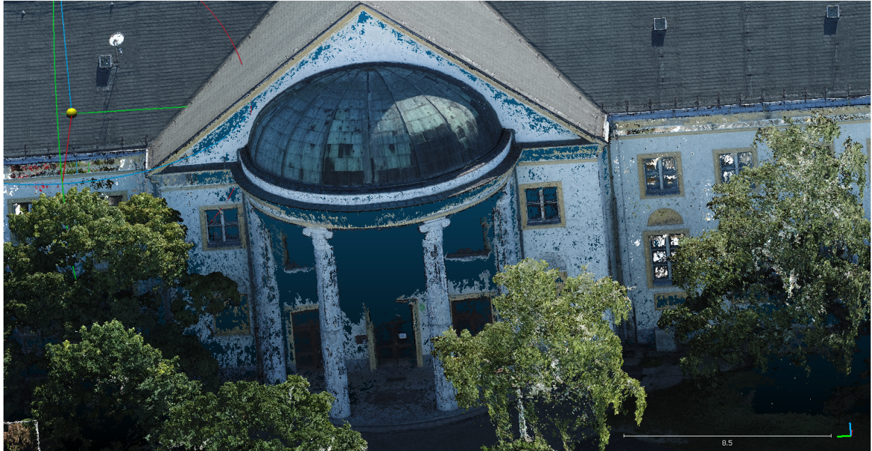
Figure 17. The focus area of the western facade of the building as seen in the DJI Phantom 4 Pro point cloud
