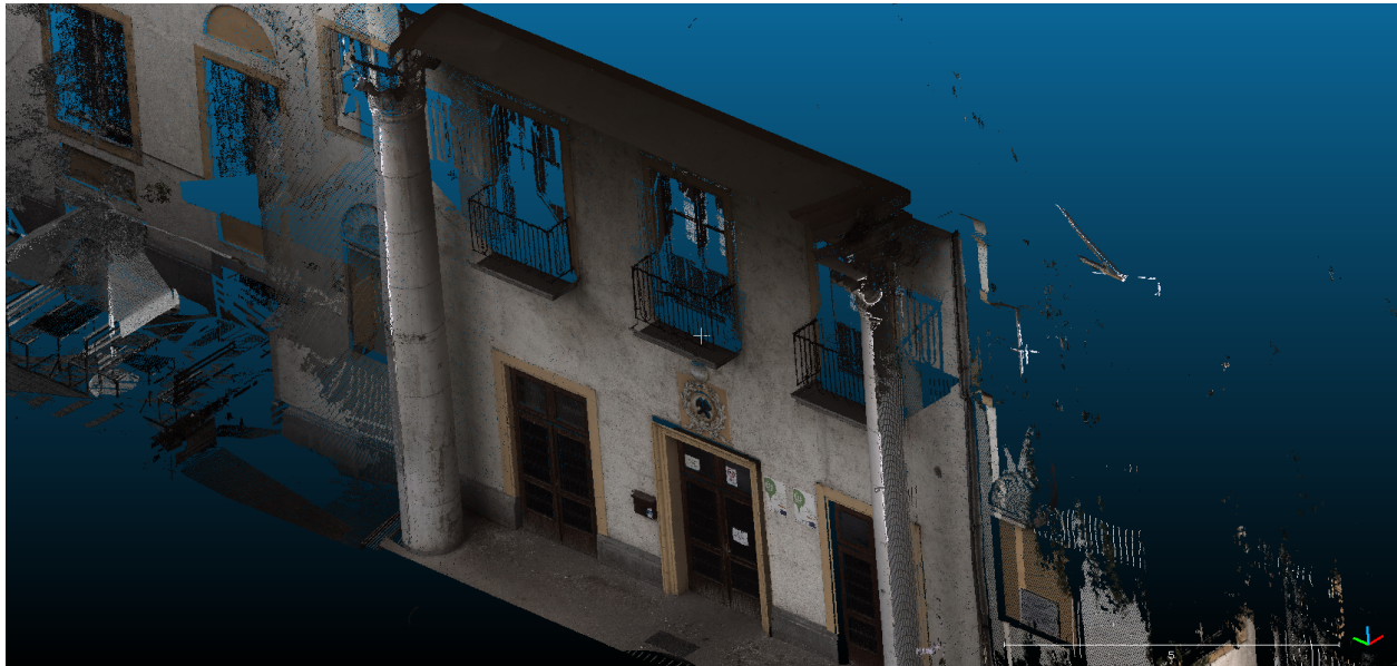
Figure 28. The view of the facade that offers a better perspective over balconies and their railings as seen in the Leica P40 point cloud (RGB)
