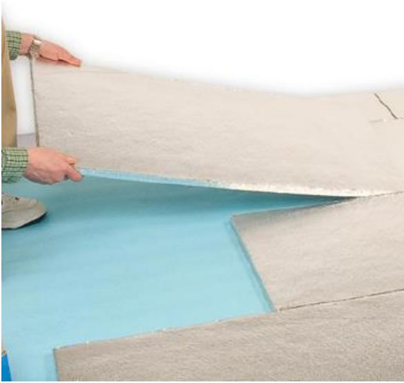
Figure 10 VIPs being installed [86]
