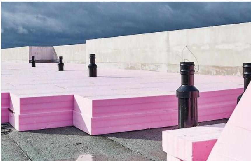
*Figure 7 XPS roof insulation while installation [23]*
