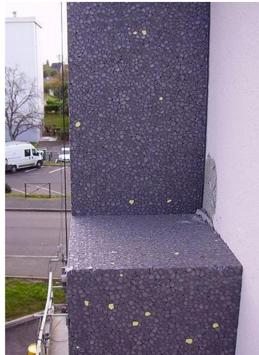
*Figure 6 EPS insulation while installation [82]*
