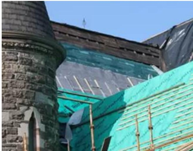
Figure 11 Aerogel as thermal insulation while renovating historical buildings [49]
