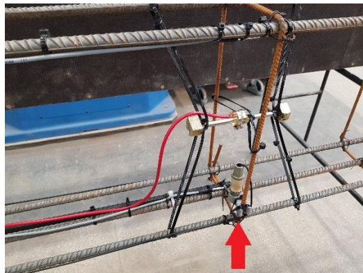
Figure 11- Example of Installation of strain sensor
