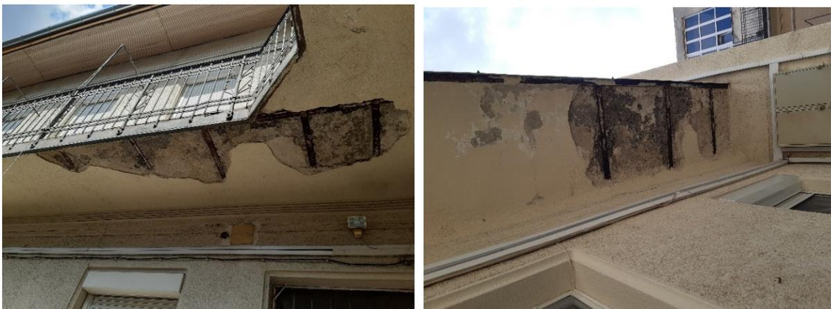
Figure 8.a,b Material loss, illustrated on the bottom part of the balconies
