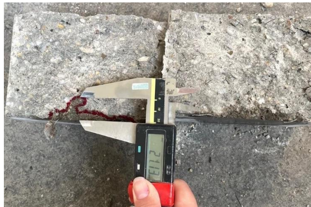
Figure 5.5.5 – Water permeability test, specimen split open
